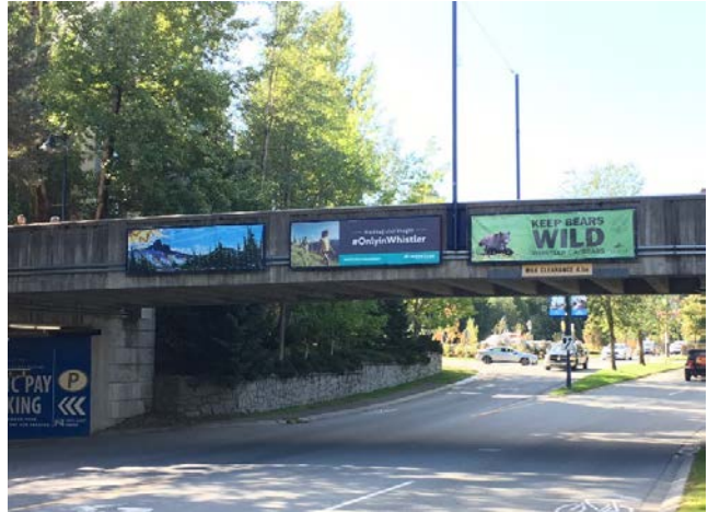
Ted Nebbeling Bridge East
